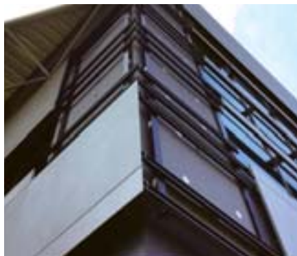
Cut-To-Size Slabs Installed onto the Highly Engineered Sub-Frame and Adhered to the Extruded Aluminum Profiles with Structural Silicon
