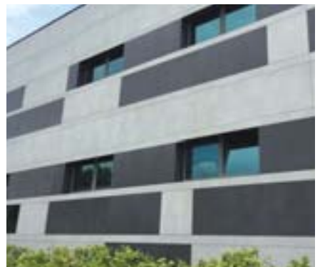
Cut-To-Size Slabs Installed onto the Highly Engineered Sub-Frame and Adhered to the Extruded Aluminum Profiles with Structural Silicon
