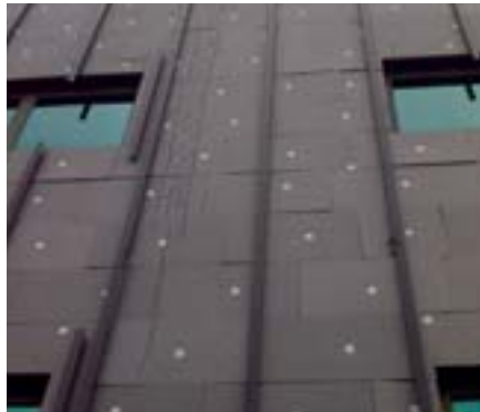
Installation of Ridged Insulation, Vertical T-Profiles, and Horizontal Rails
