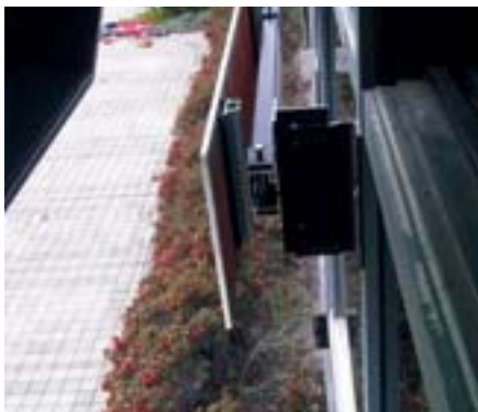
Cut-To-Size Slabs Installed onto the Highly Engineered Sub-Frame and Adhered to the Extruded Aluminum Profiles with Structural Silicon
