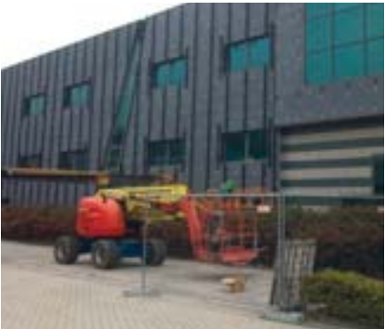
Installation of Ridged Insulation, Vertical T-Profiles, and Horizontal Rails
